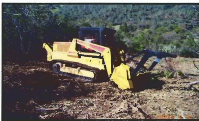
Small masticator used on smaller acreage. Equipment on tracks for minimal soil disturbance. Note the drum head attachment for “chewing up the vegetation.”
